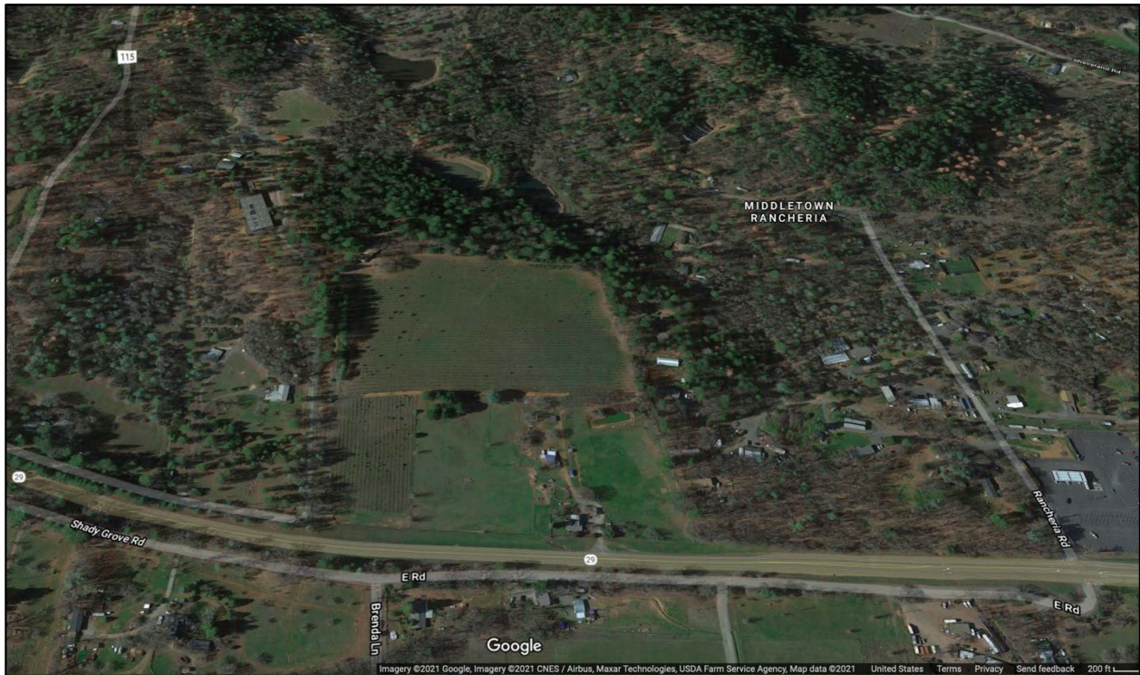
Figure 2.3.2. Oblique aerial photo, view looking west, of subject property and surrounding properties (Google Maps).
